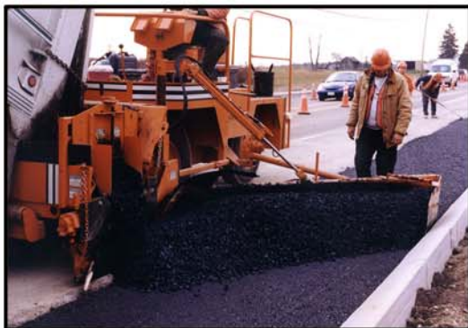
SPD spreading with LEFT HAND BLADE, after a QUICK change over from the right side.
